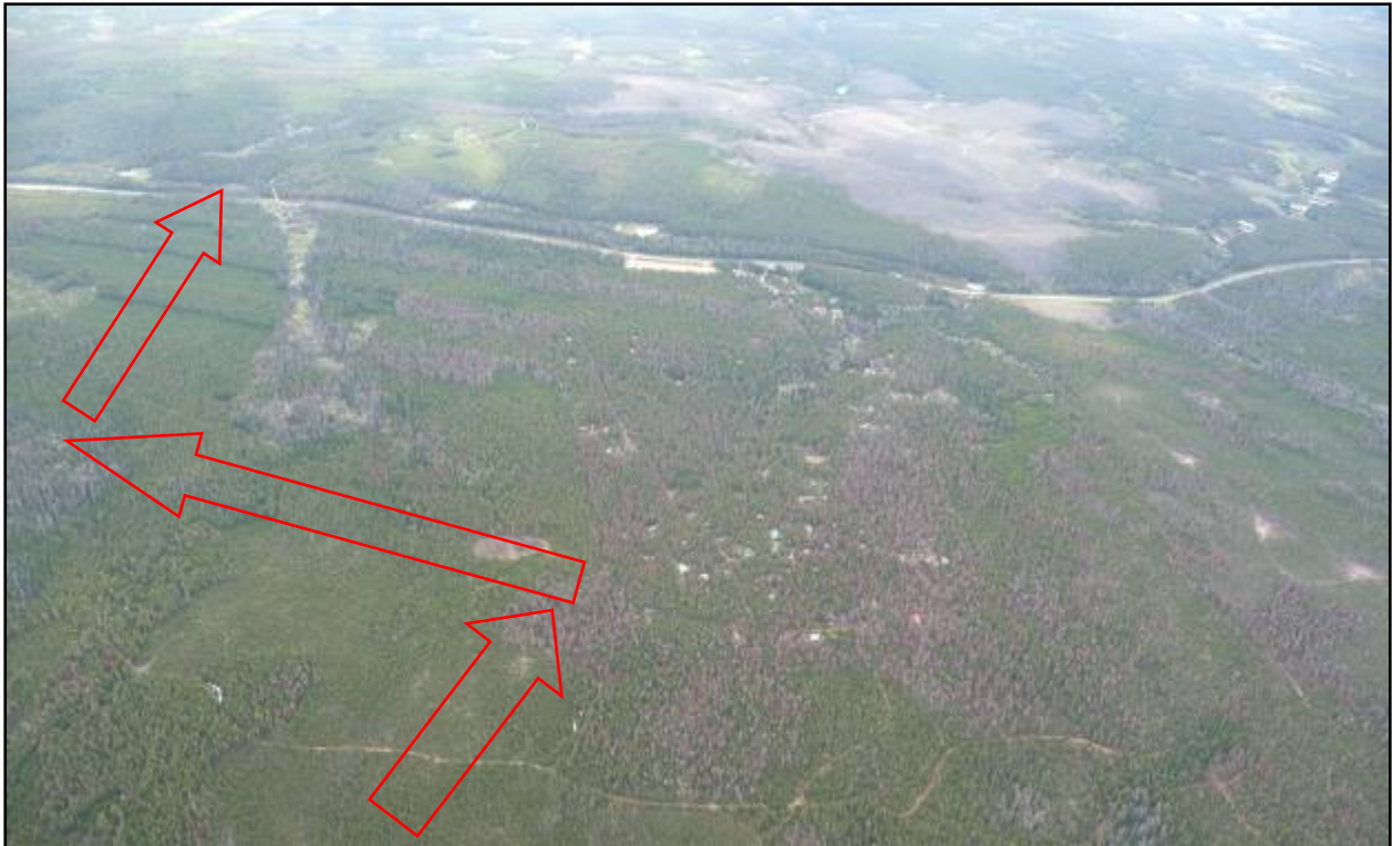
Photo 12. M56 bumps into a small subdivision and skirts around it and across WY Hwy 230.
